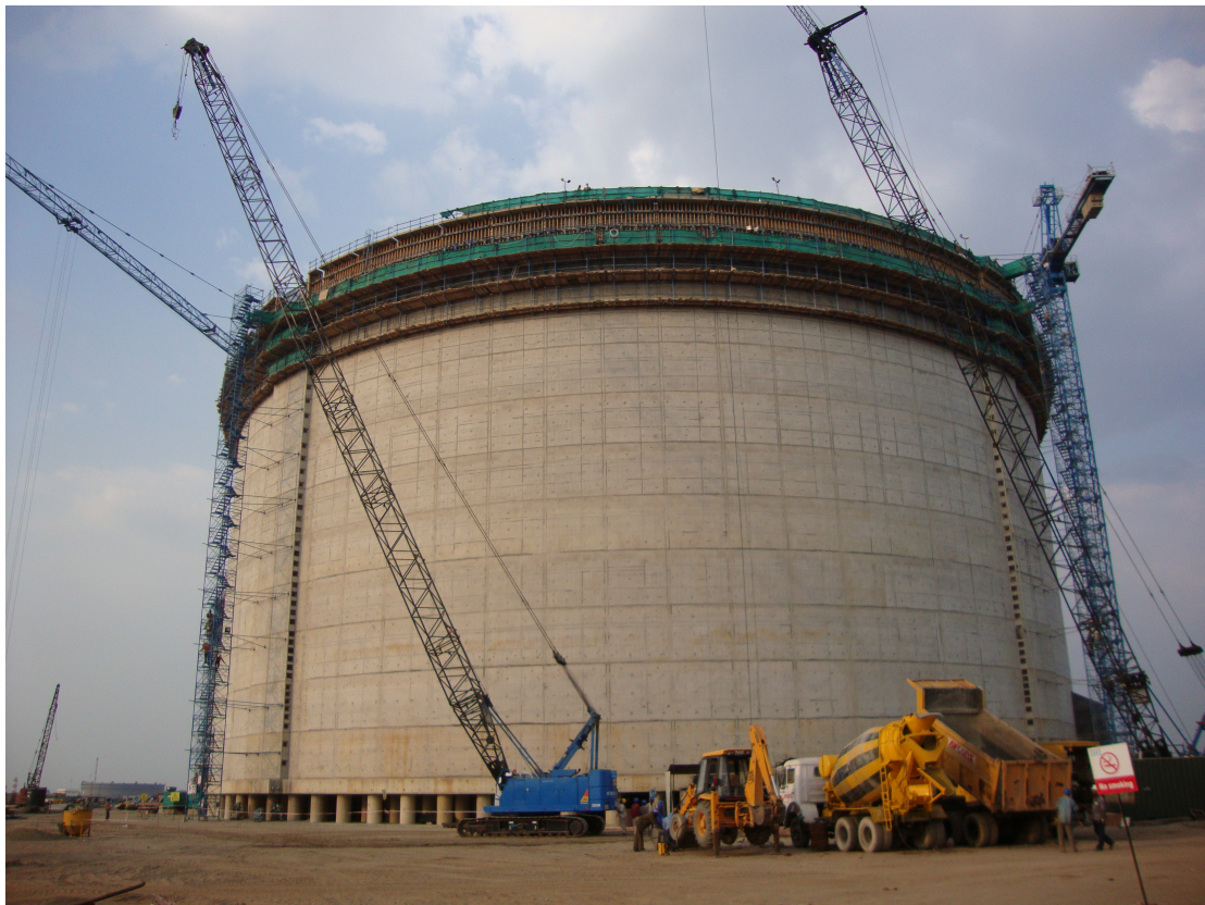
Completed view of tank
